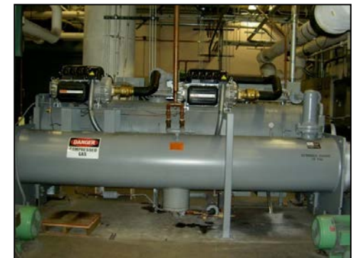
Compressor Retrofit at San Diego – Two Compressors
