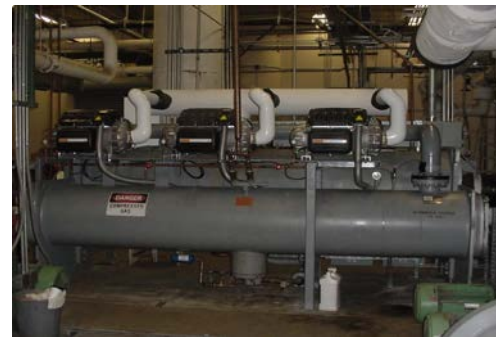
Compressor Retrofit, San Diego – Three Compressors
