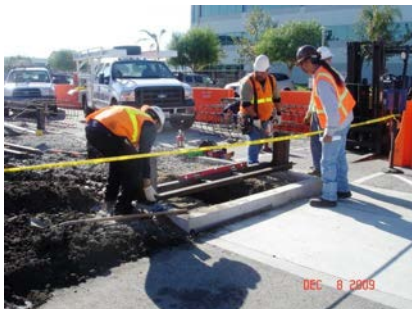
Construction of PV Parking Canopy Los Angeles AFB
